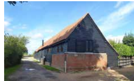
Figure 58: Barn at Burge End Farmhouse
