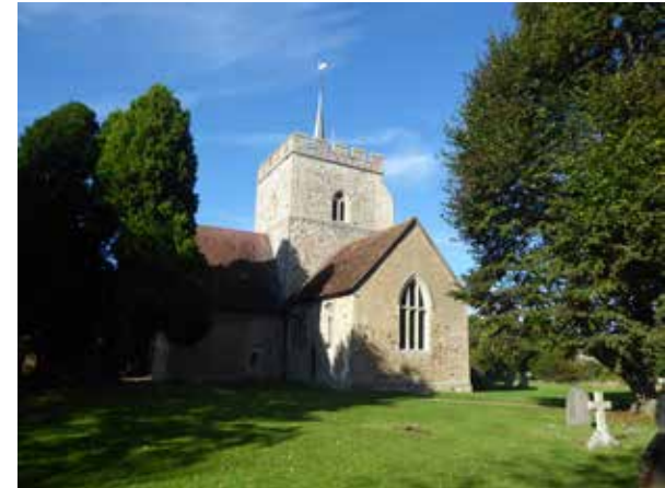
Figure 31: St Mary's Parish Church
