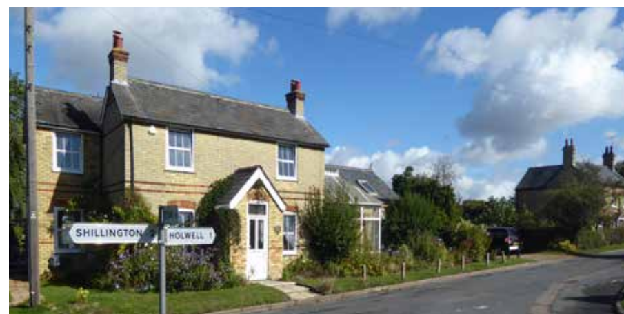
Figure 19: Houses on Holwell Road which are proposed to be added to the Conservation Area
