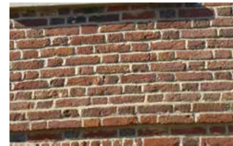
Figure 43: Example of Flemish bond brickwork with imperial bricks
