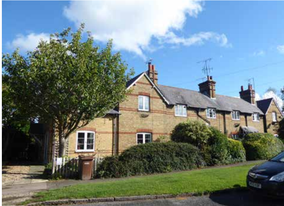
Figure 23: Nineteenth century cottages on the High Street, built in local Arlesey white brick with decorative red brick banding
