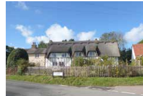
Figure 36: 4-6 Walnut Tree Road
