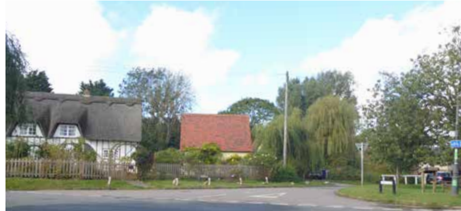
Figure 107: Poorly proportioned modern outbuildings detract from the appreciation of their host dwellings
