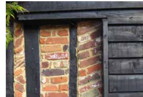
Figure 42: Example of exposed brick nogging
