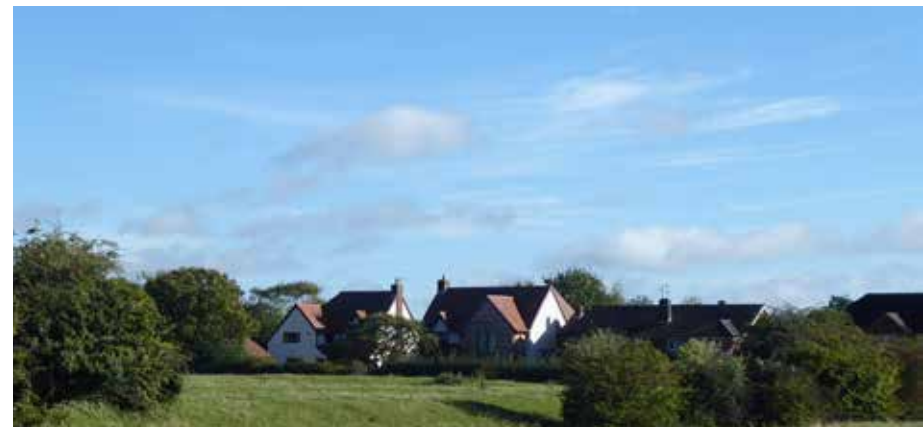
Figure 108: An example of where recently altered dwellings are prominent due to their incongruous height and material choice
