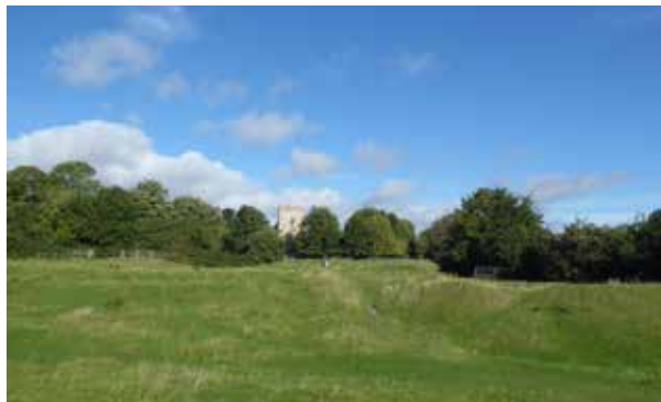
Figure 27: Earthworks in The Bury, with St Mary's Church behind
