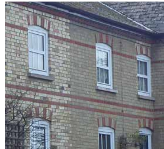
Figure 61: An example of where modern uPVC windows have been installed to replace wooden sashes
